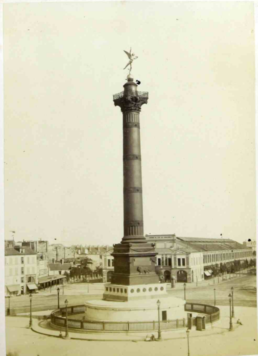
Column of the Regeneration
